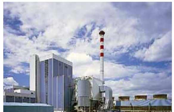
Edenderry Power Station.
