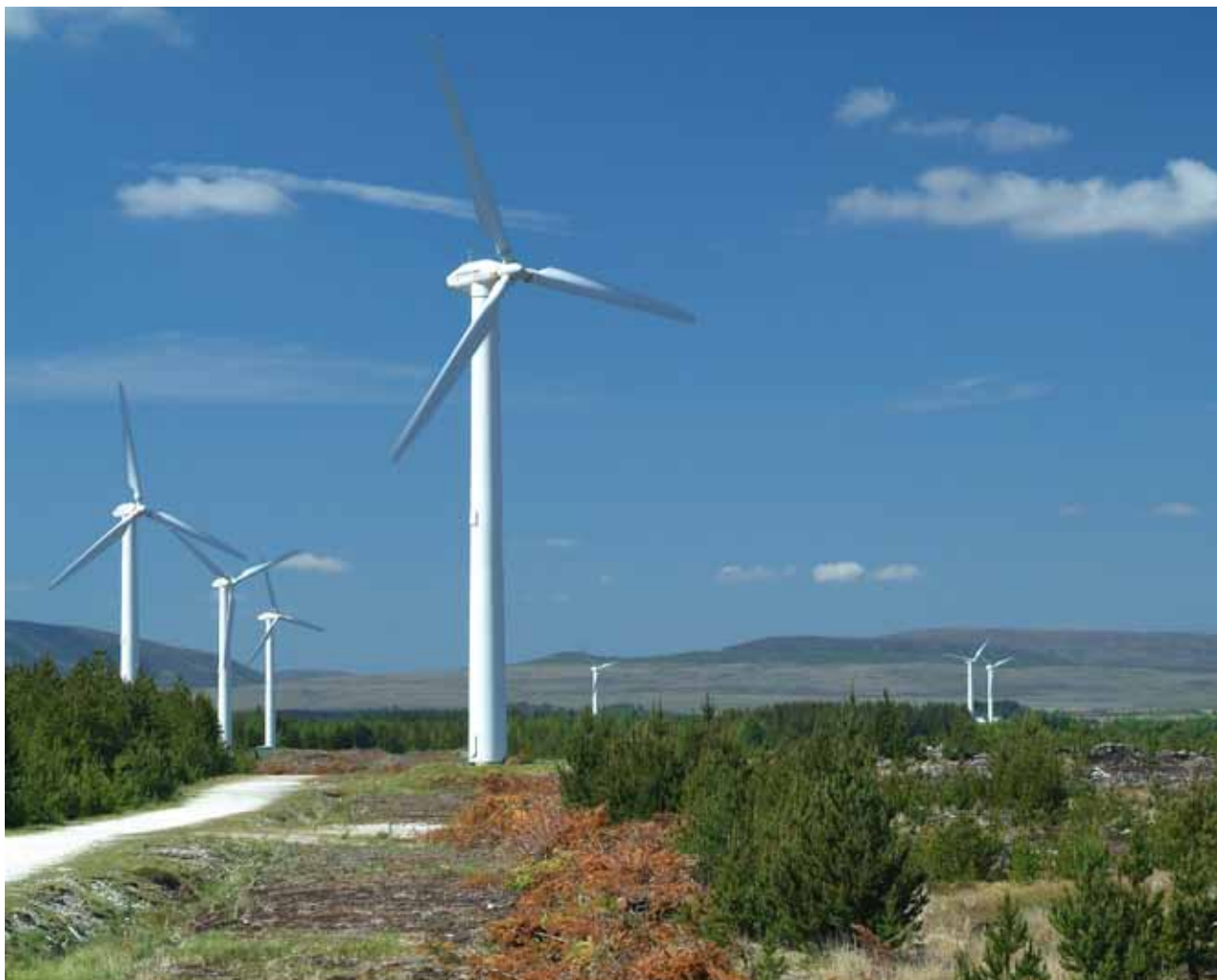
Wind turbines at Oweninny Wind Farm.
